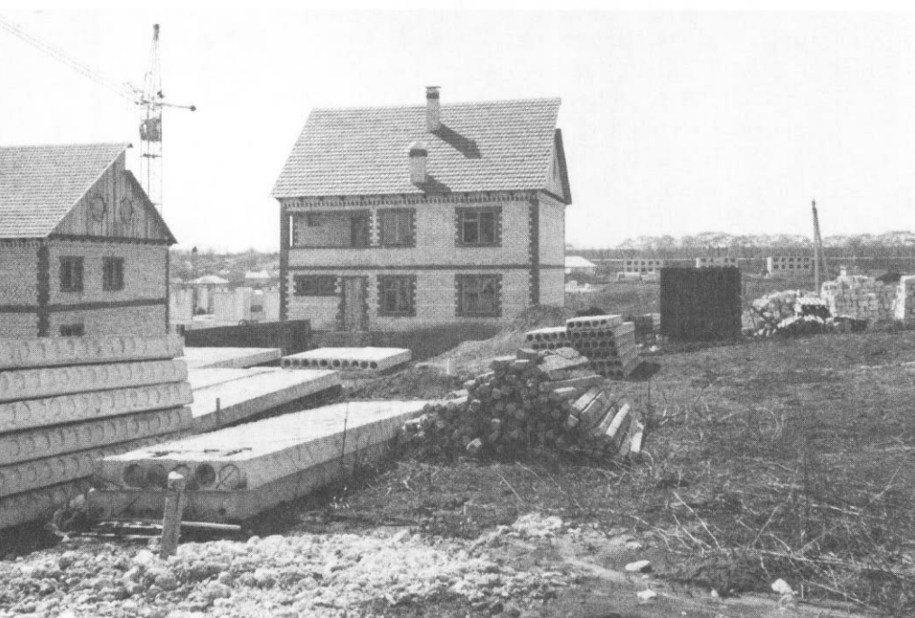
Sunday afternoon flower market, Chisinau Courtesy Tom Skipper Private housing under construction, Stauceni Courtesy Charles King
